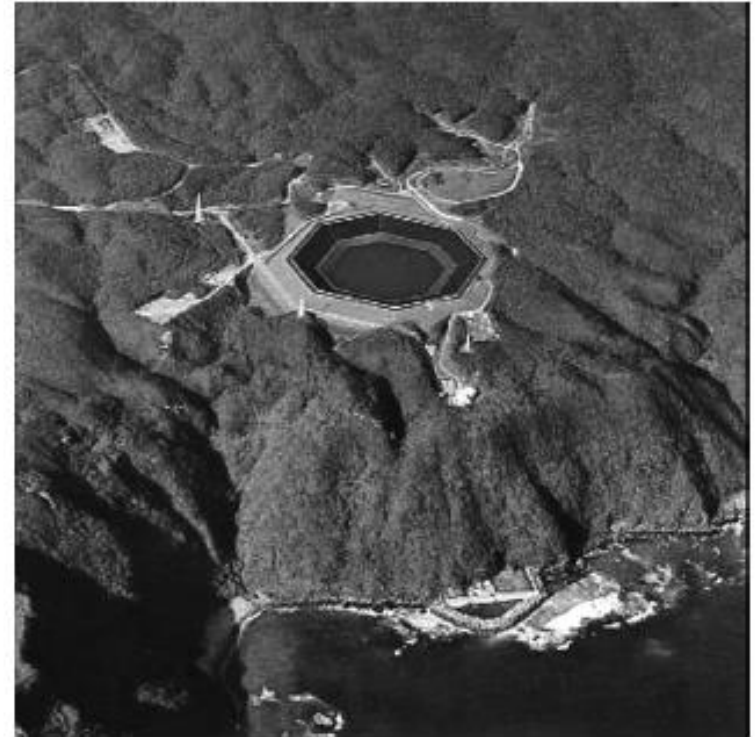
Fig. 10.5 The Okinawa pumped storage plant in Japan. Source: Agency of Natural Resources and Energy Japan.
